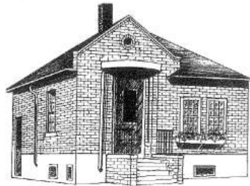
28) 610 Varennes Street: The location of Wolseley's Town Office since 1963, this building was designed in 1937 as the local "Telephone Exchange" by the Regina architectural firm Storey and Van Egmond. It was originally faced with Ruff-Text brick made at Claybank but, with an addition to the east, the front was stuccoed to present a continuous construction material on the south and east façades. The original brick is still visible on the west side.
